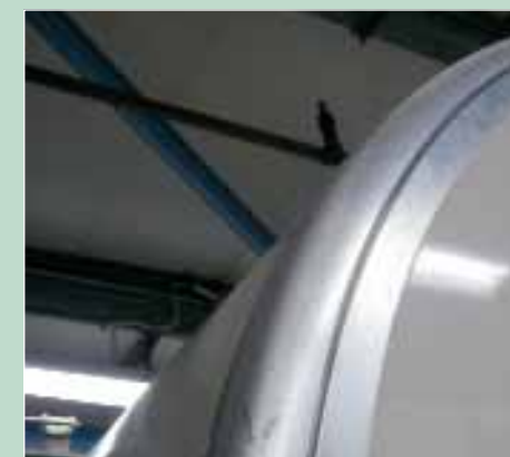
Bailey found a specialist that could curve these structural frame members
